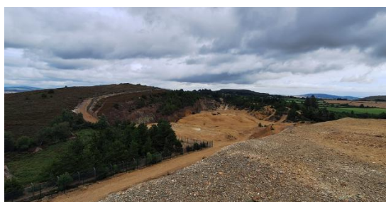
New perimeter fencing at Avoca Mines East
